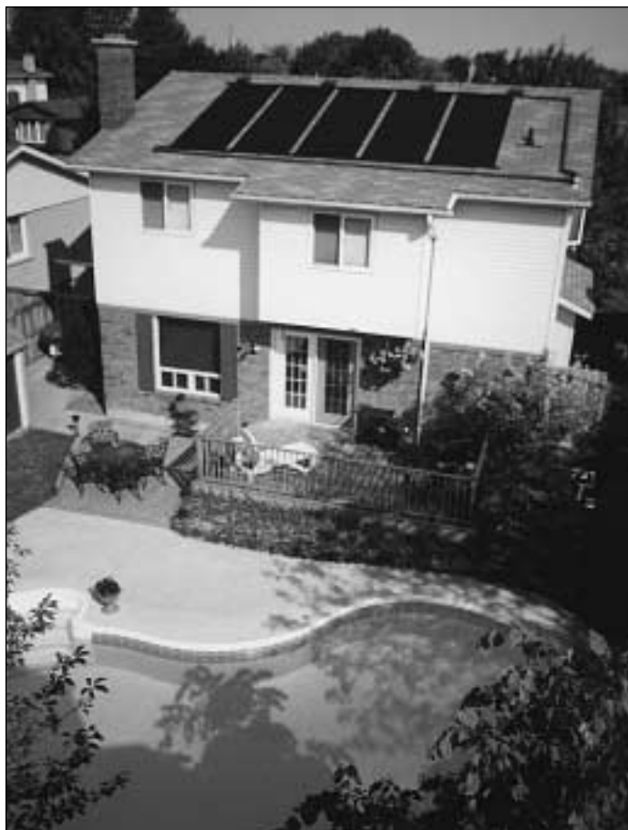
Roof-mounted solar collectors are used to heat the pool below, reducing energy costs.
